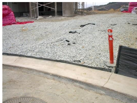
Good application of rock exit pad. Note short section of material against curb that is keeping rock from leaving site. Photo credit: John Kosco, Tetra Tech.
