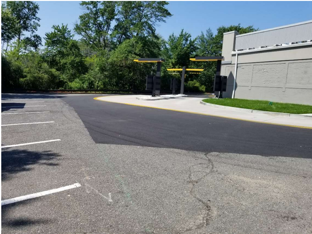
Photo 4 – Photo of the drive-thru lane facing the southern property line of the site.
