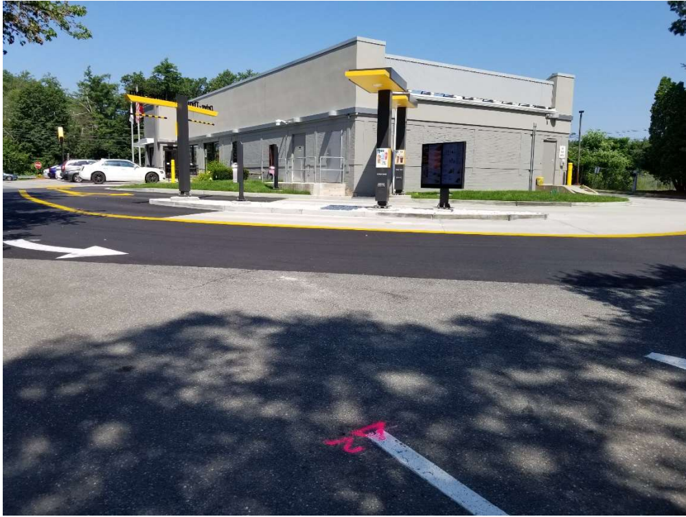
Photo 3 – Photo of the drive-thru lane facing the rear of the building.
