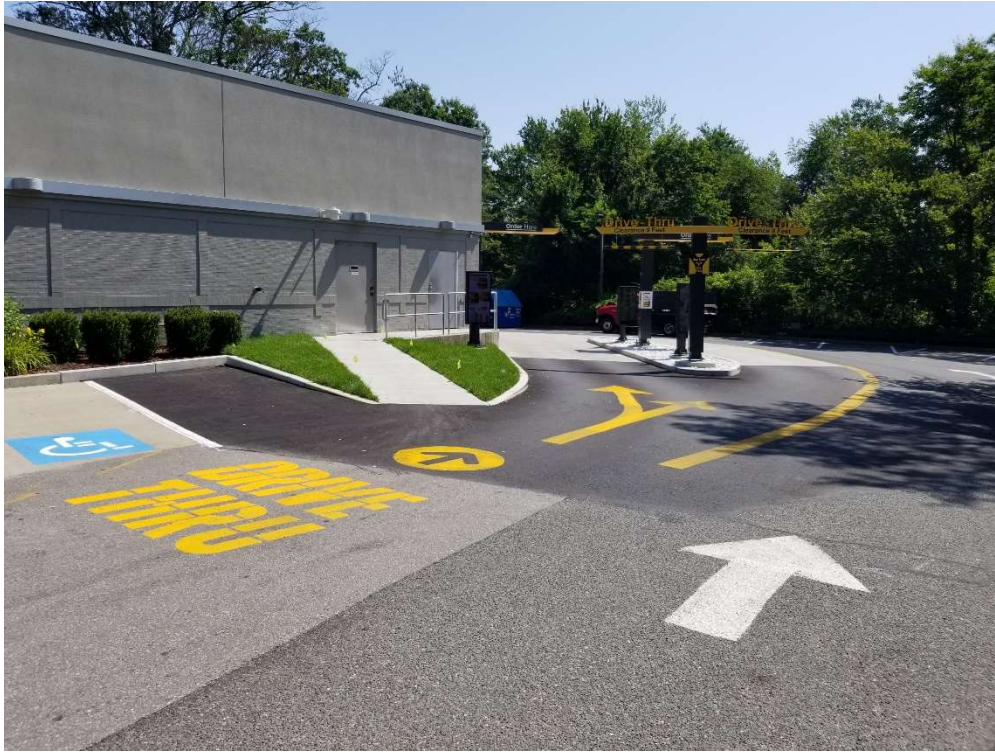
Photo 1 – Photo of the drive-thru lane facing east toward the rear portion of the site.
