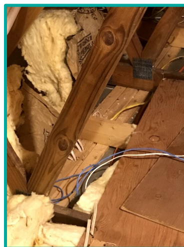
Attic – Insulation Void
