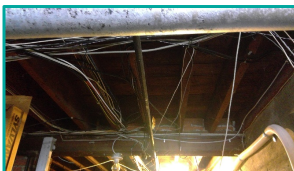
No insulation in basement ceiling
