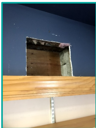
Evidence of Wall Insulation
