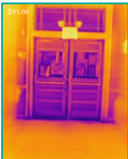
Entry door with transom window – thermal image
